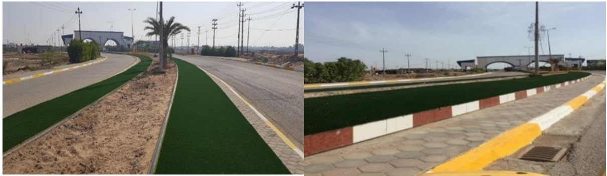
Picture 17: Phase 3 - Faw entrance road & Corniche street
