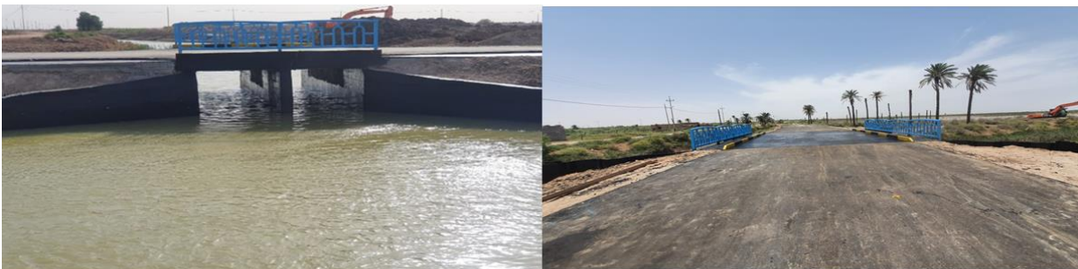
Picture 18: Phase 3 - Steel structure bridge
