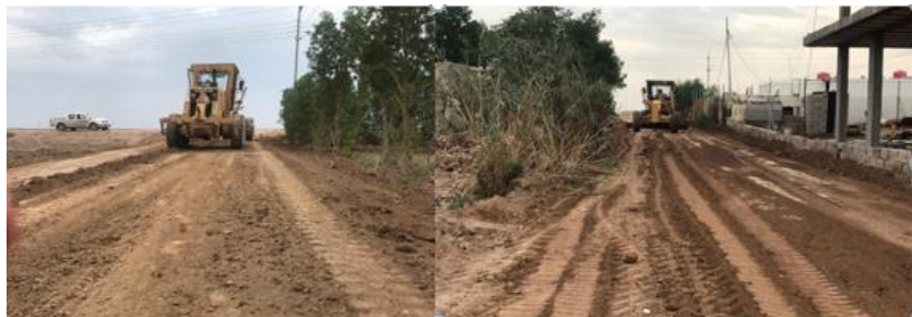
Picture 19: Phase 4 - Siba Project - 15 KM Roads Construction in progress
